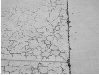
Extrusion of joint-sealants
